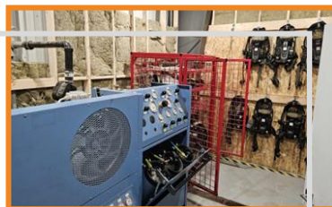
Compressor / Storage Room
