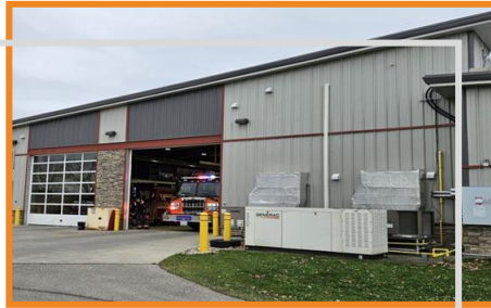
Back of Station
