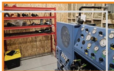
Compressor / Storage Room
